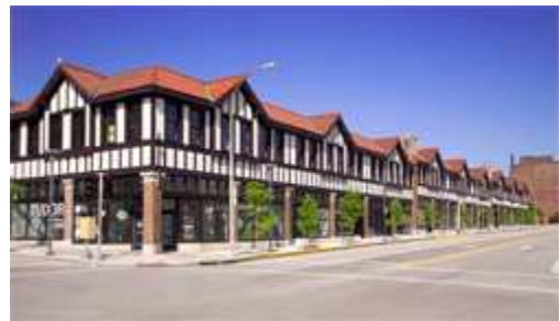
Tudor Building after rehabilitation
