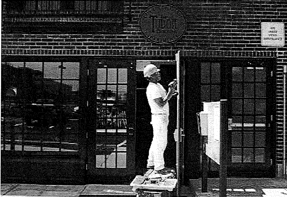
The Tudor Building is a mix of retail spaces and affordable apartments in downtown St. Louis. Tom Luechtefeld, a carpenter with Paric Corporaton puts the finishing touches on a door at The Tudor Building located in the 1900 block of Washington Avenue.
